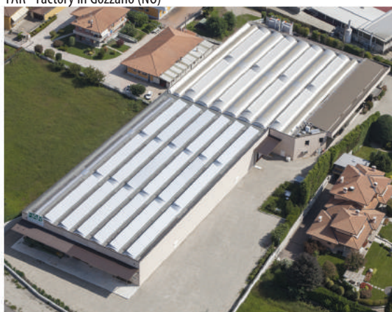
FAR - New factory in Gozzano (NO)
